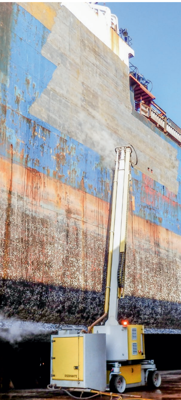
Dockmate - ship cleaning system
