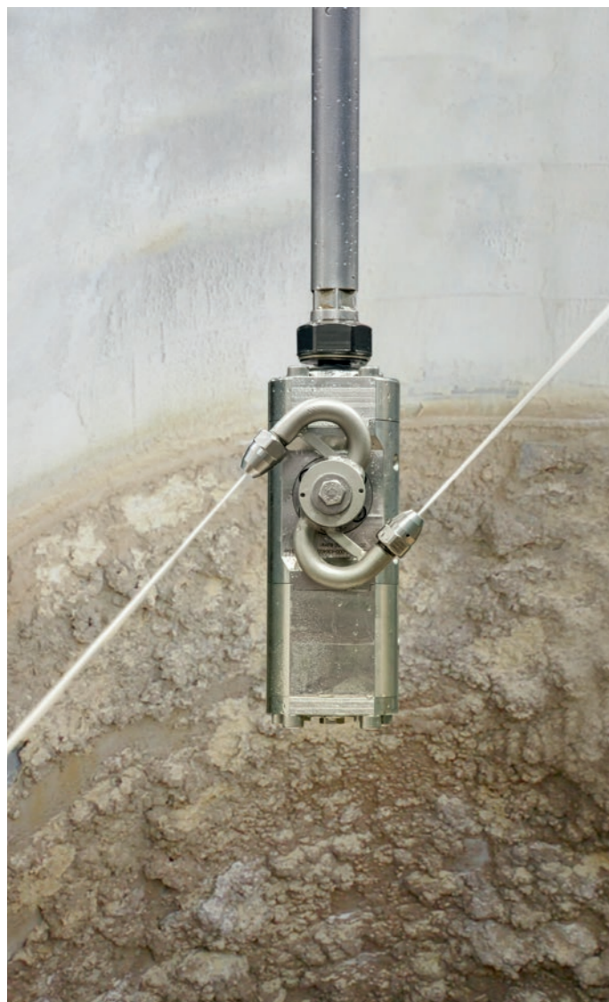
Aquamat - Tank cleaning units
