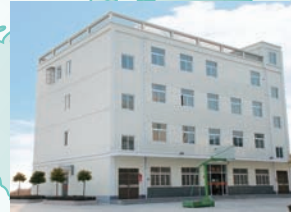
Qidong Head Office
